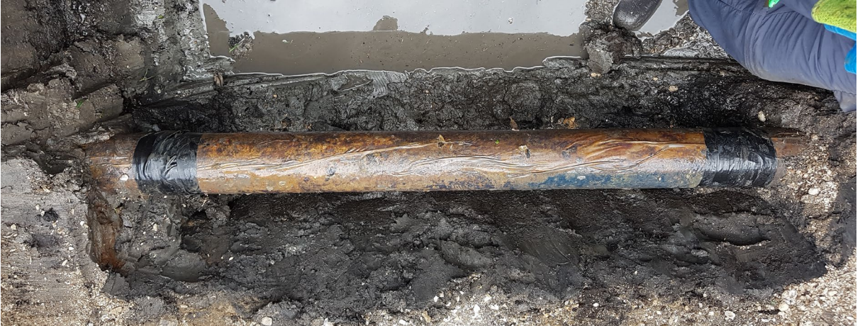
D: Site 2 - Prior to removal of polyethylene film
