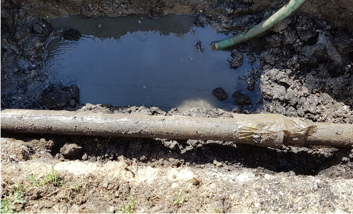
A: Pipe exposed prior to removal of polyethylene film
