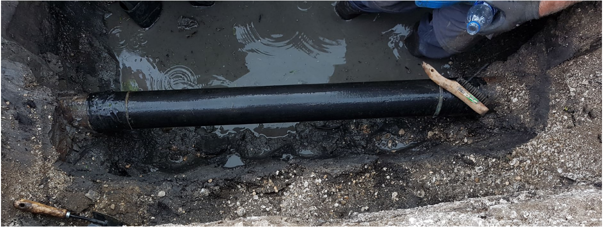
F: After cleaning and sounding of the pipe surface
