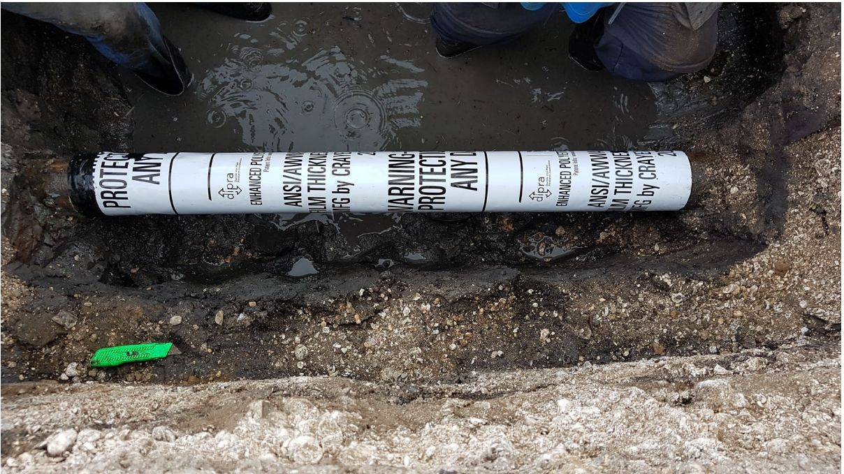
G: Pipe encased in V-Bio ® enhanced polyethylene encasement prior to backfilling
