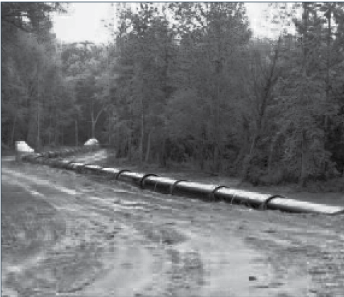
Above: Ductile Iron Pipe is utilized for innovative solutions of sewerage piping problems. Illustrated is an “at grade” gravity sewer.
