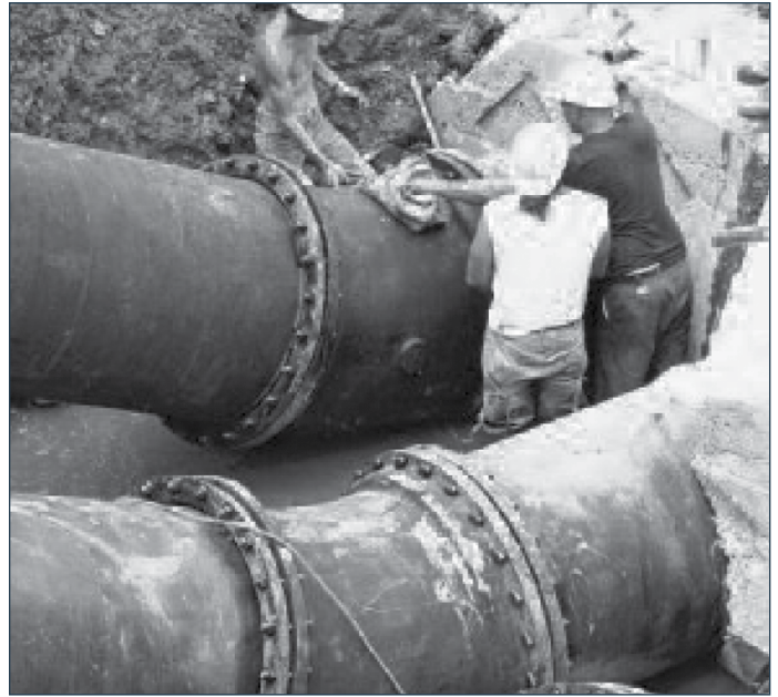
Ductile Iron Pipe is often used for inverted siphons in difficult installations such as the stream crossing shown here because of its great strength, joint integrity, and its versatile and readily available joints and fittings.
